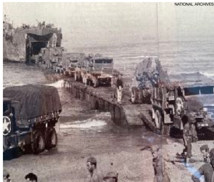
First used during the Sicily invasion, trucks loaded with supplies drive from LST-336. Pontoon causeways were used widely in the Atlantic and Pacific theaters.
